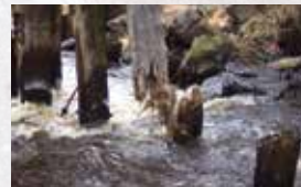
Broken bridge trestle along the Willard Munger State Trail (©Minnesota DNR)
