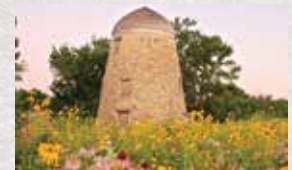
Historic Seppman Mill in Minneopa State Park is in need of repairs (©Randy Wood)
